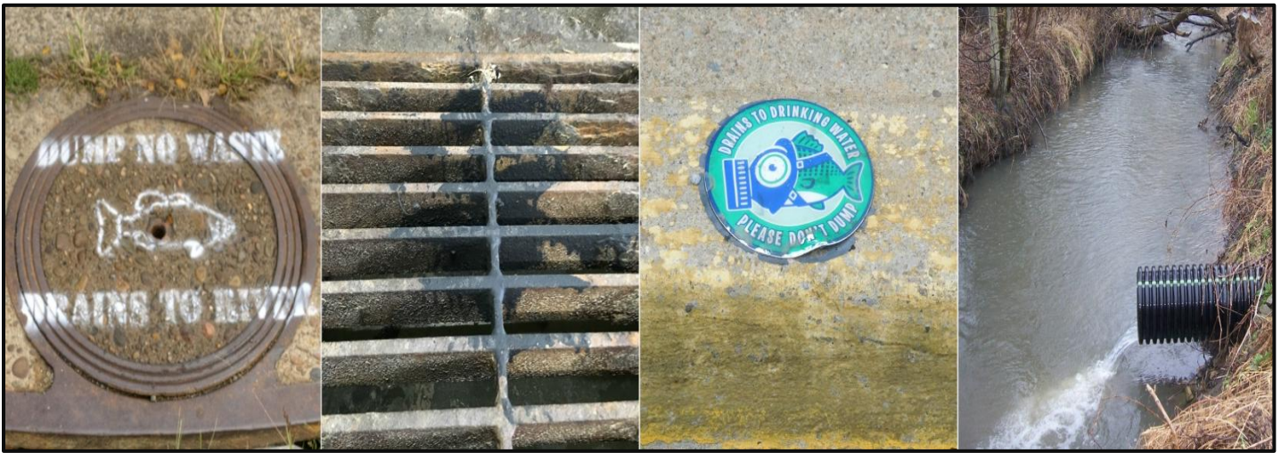
Figure 6: From left to right: A stenciled storm drain in Pittsburgh; Staining which shows some sort of illicit discharge poured down a drain; A "no dumping" stormwater identification marker in Etna; An outfall to a stream (Sources: SPC and Westmoreland Conservation District)
