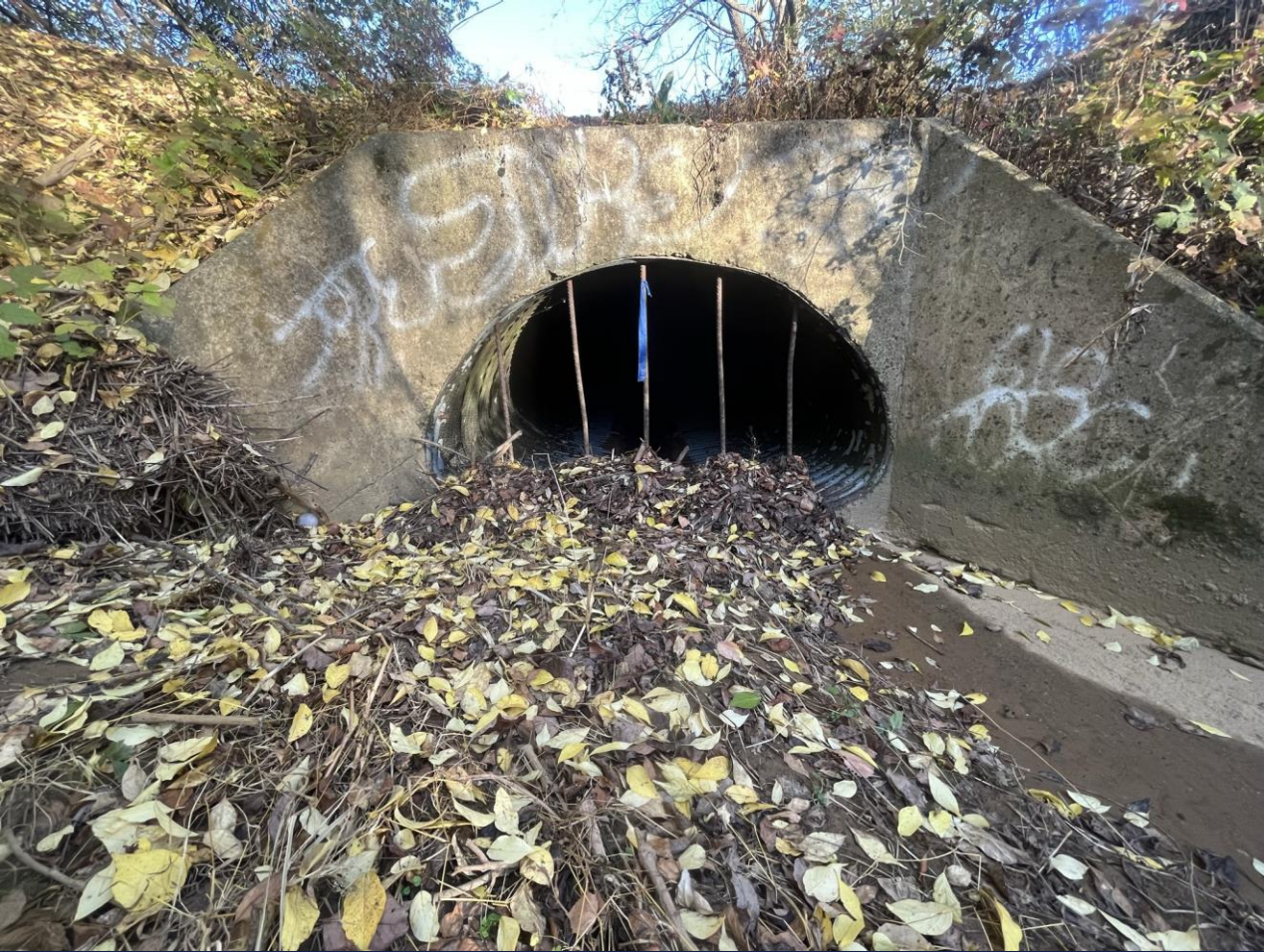
EXISTING HEADWALL FOR 72" X 44" DRAINAGE PIPE ABOVE MEADOW AVENUE
